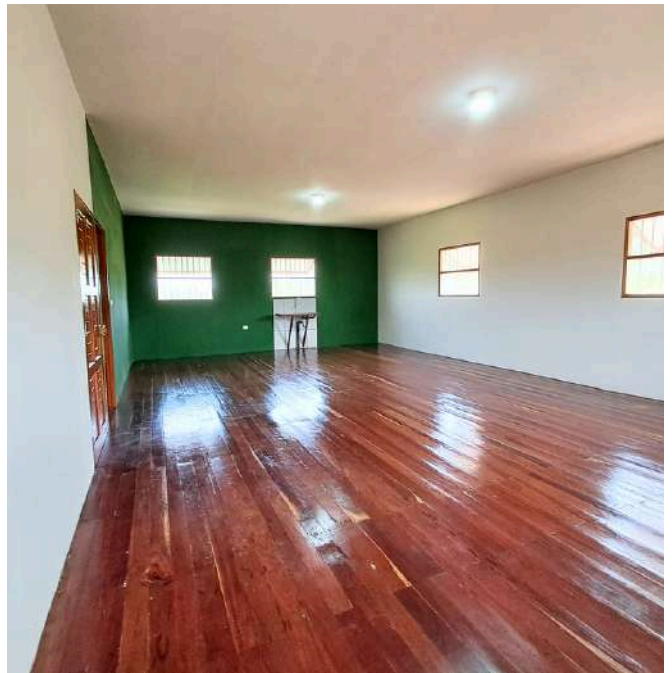
In the first half of 2025, we’ll be equipping the lab and installing solar panels
